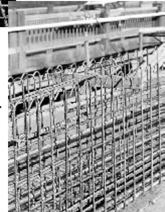
Vertical arrangement of bent stainless rebar; Haynes Inlet Slough Bridge.
